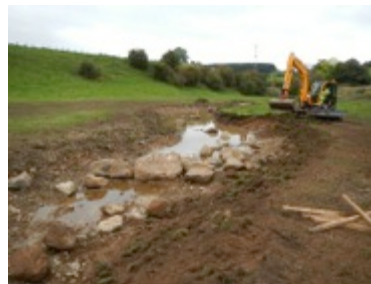
Creating the new channel for the River Leith, near Penrith
